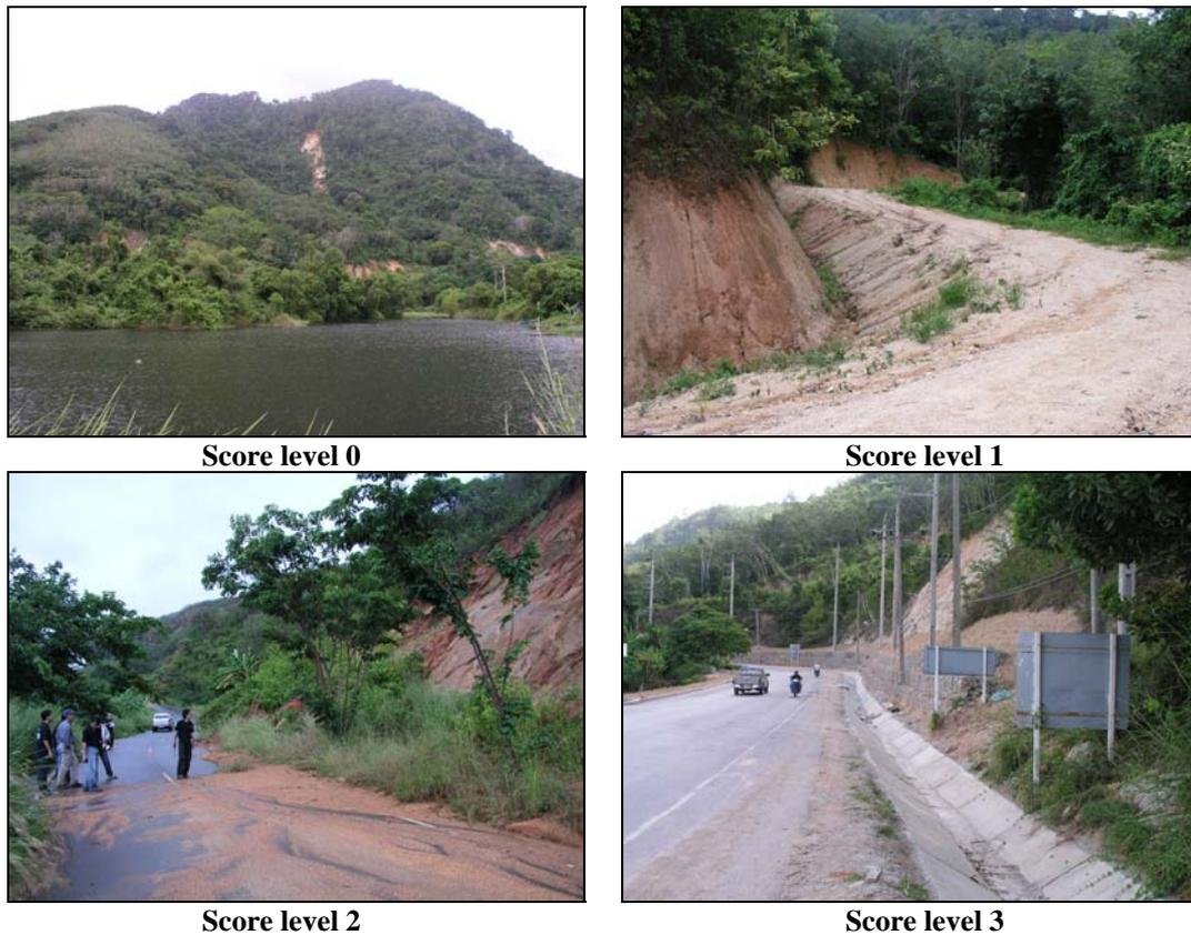
Figure 6 Example of scoring level for consequence factor of infra-structure damages
