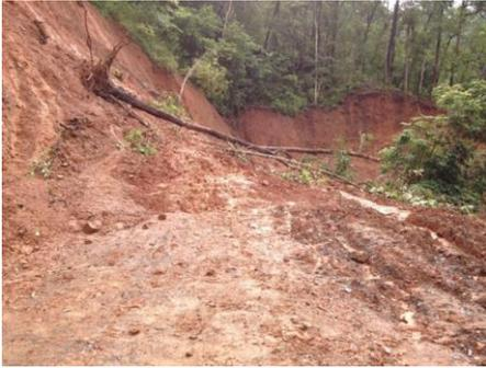
Fig. 2. Slope failure in cut slope
