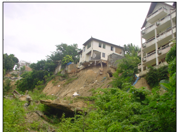
Fig. 1 Na Nai roadside landslide on October 25, 2007
