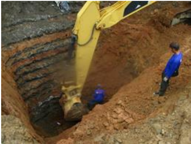
Figure 31 Roughness Surface in rehabilitation processes of Mae Suai Dam (2019)
