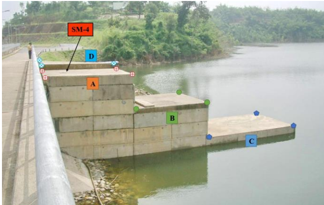
Figure 9 Reference point at surface of RCC block (Photo by RID)
