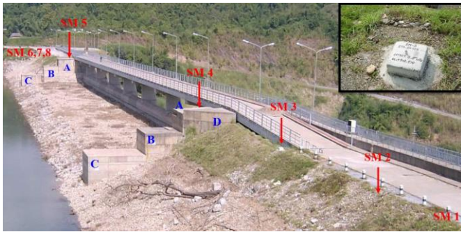
Figure 4 Spillway wing wall and Location of Surface Monument (Photo by RID)
