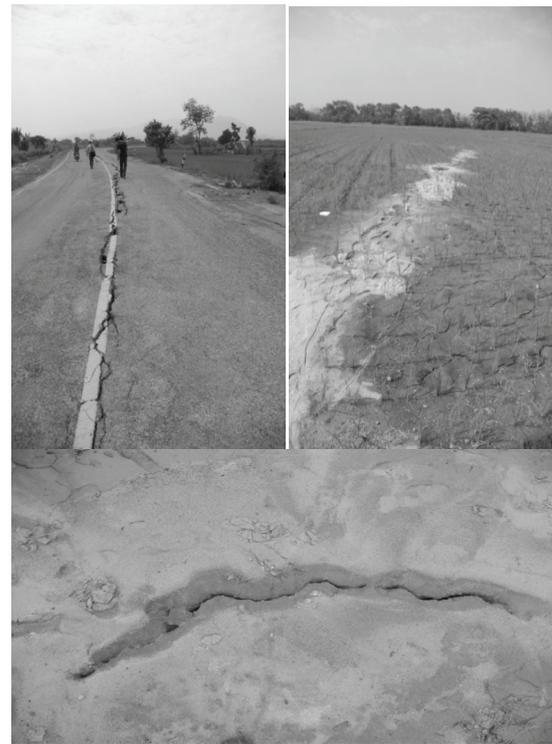
Figure 3 : Liquefaction evidences in Maesai, Chiangrai, Thailand
