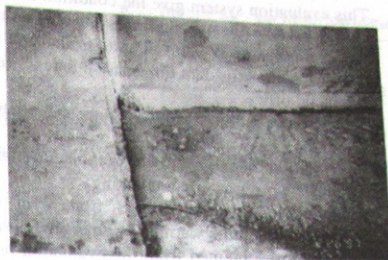
b) Piping on spillway flood
