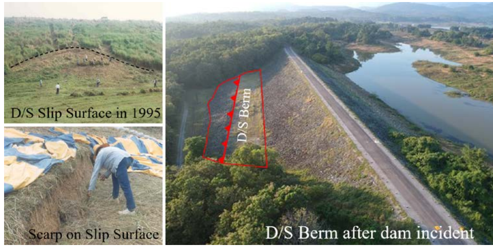
Figure 7 Dam indent on 1995 and stabilization of D/S slope by rock berm
