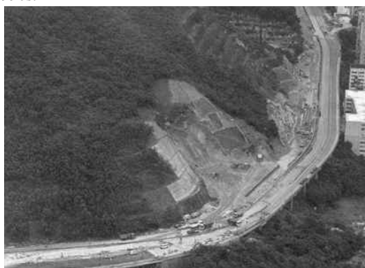
Figure 2: The Ching Cheung Road Landslide in 1997
