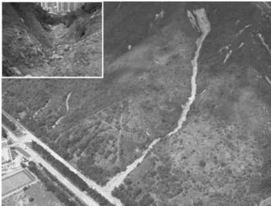
Figure 5: Yu Tung Road channelized debris flow
