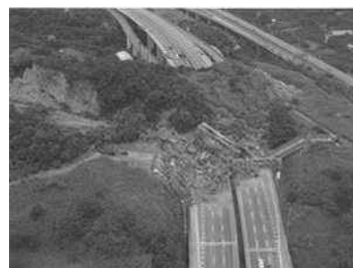
Figure 1. National Highway No. 3 at 3.1k accident
