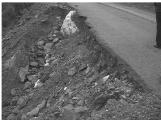
Figure 1. Photo of local slope failiures
