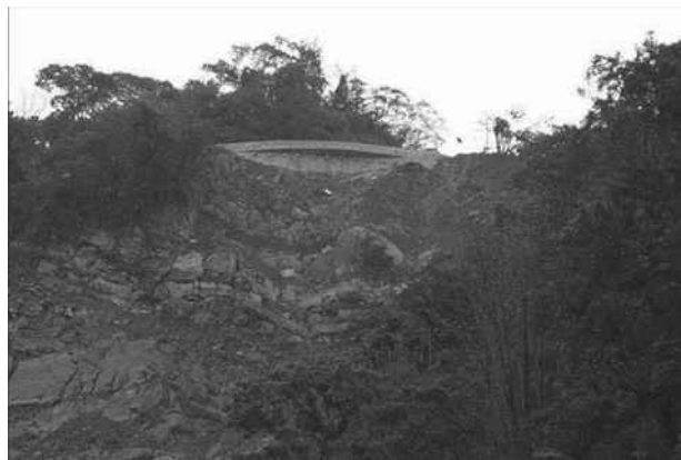
Figure 7. Completion of box-type structure at Mileage 39Km.
