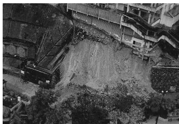
Figure 1: The Kwun Lung Lau Landslide in July 1994
