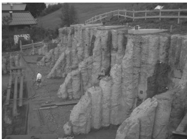
Figure 6. View of excavated MIP-walls
