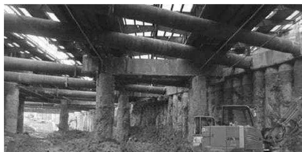
Figure 12. Picture of support beam.
