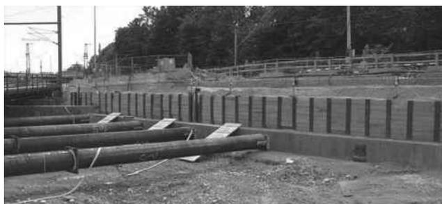
Figure 9. Encastered soldier pile wall.
