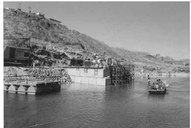
Each operation of block launching consisted of placement of blocks in the bottom course, to be followed by blocks in upper course. Till they were placed upto the level of 193.50 M. The launching of blocks is shown in photograph above.
