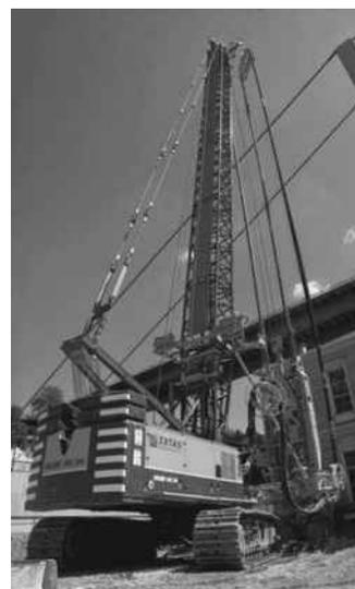
Figure 8. Diaphragm Wall Machine, Hydrofraise-Cutter
