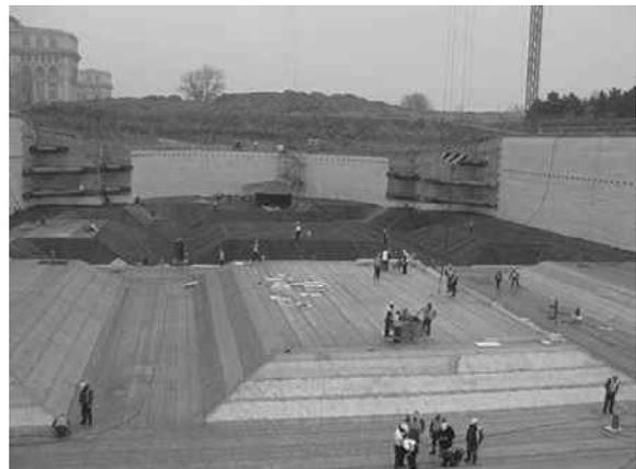
Figure 9. Lead waterproofing
