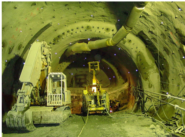
Excavation beneath Pipe Roof
