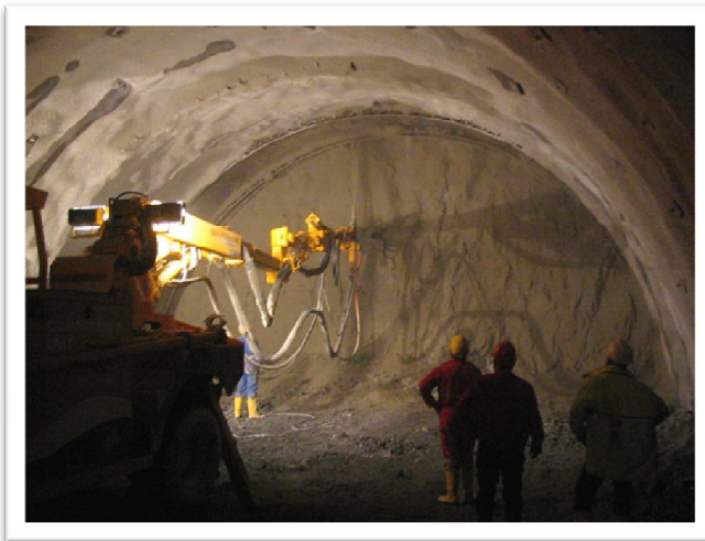
SHOTCRETE FACE SEALING
