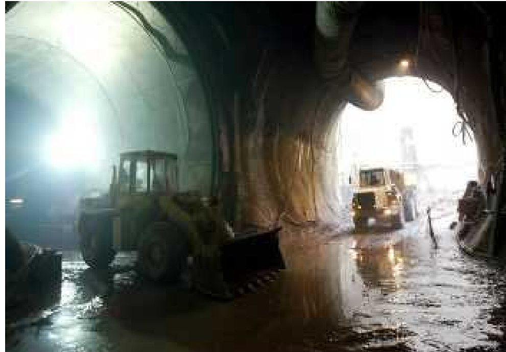
Lainzer Tunnel - Cross Passage
