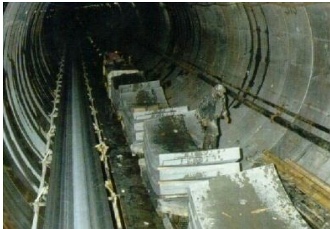
Boston Harbour Outfall Tunnel
