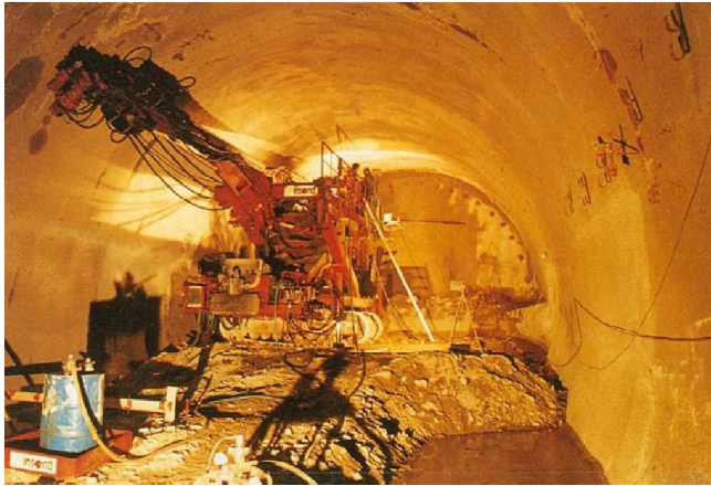
Horizontal Jet Grouting
