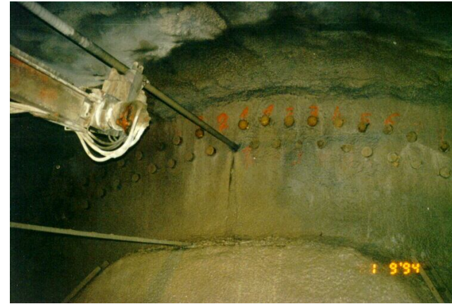
Roof Pipe Installation
