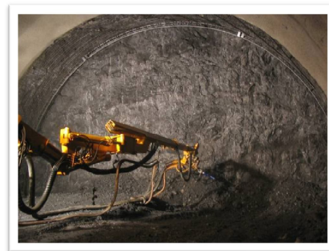
HARD ROCK FACE DRILLING
