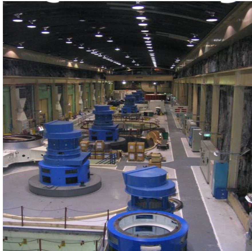
View of Manapouri Powerstation machine hall in February, 2005.
