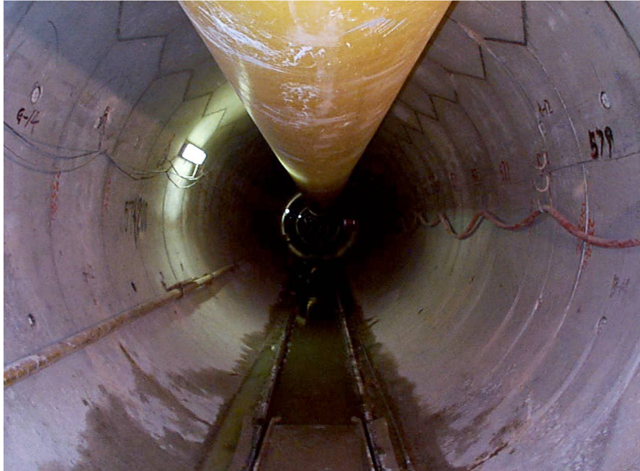
View of finished tunnel with flat joint design (WYRDPC)
