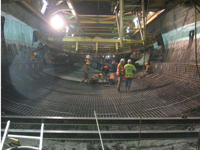
Invert Reinforcement
