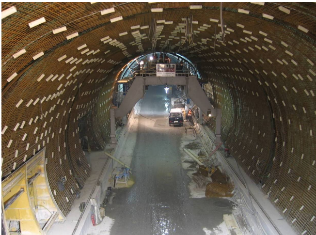
Final Lining Reinforcement
