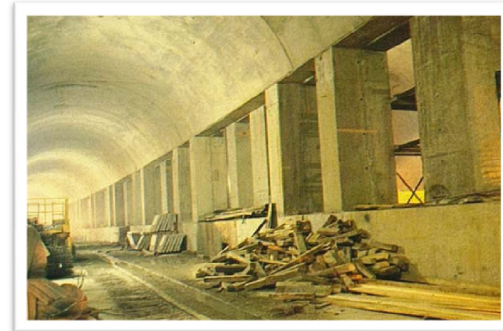
STATION TUNNEL FINAL LINING
