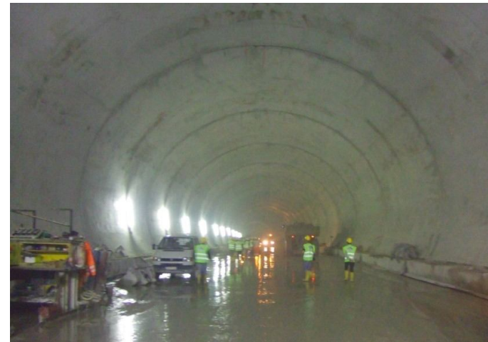
Structural Completed Tunnel
