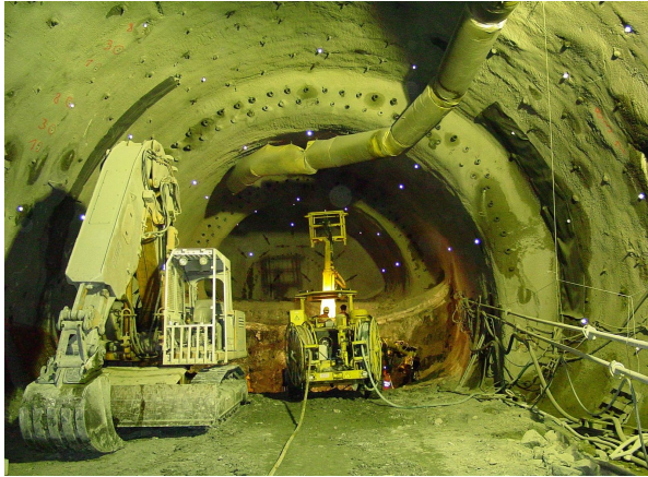
Backhoe and Shotcrete
