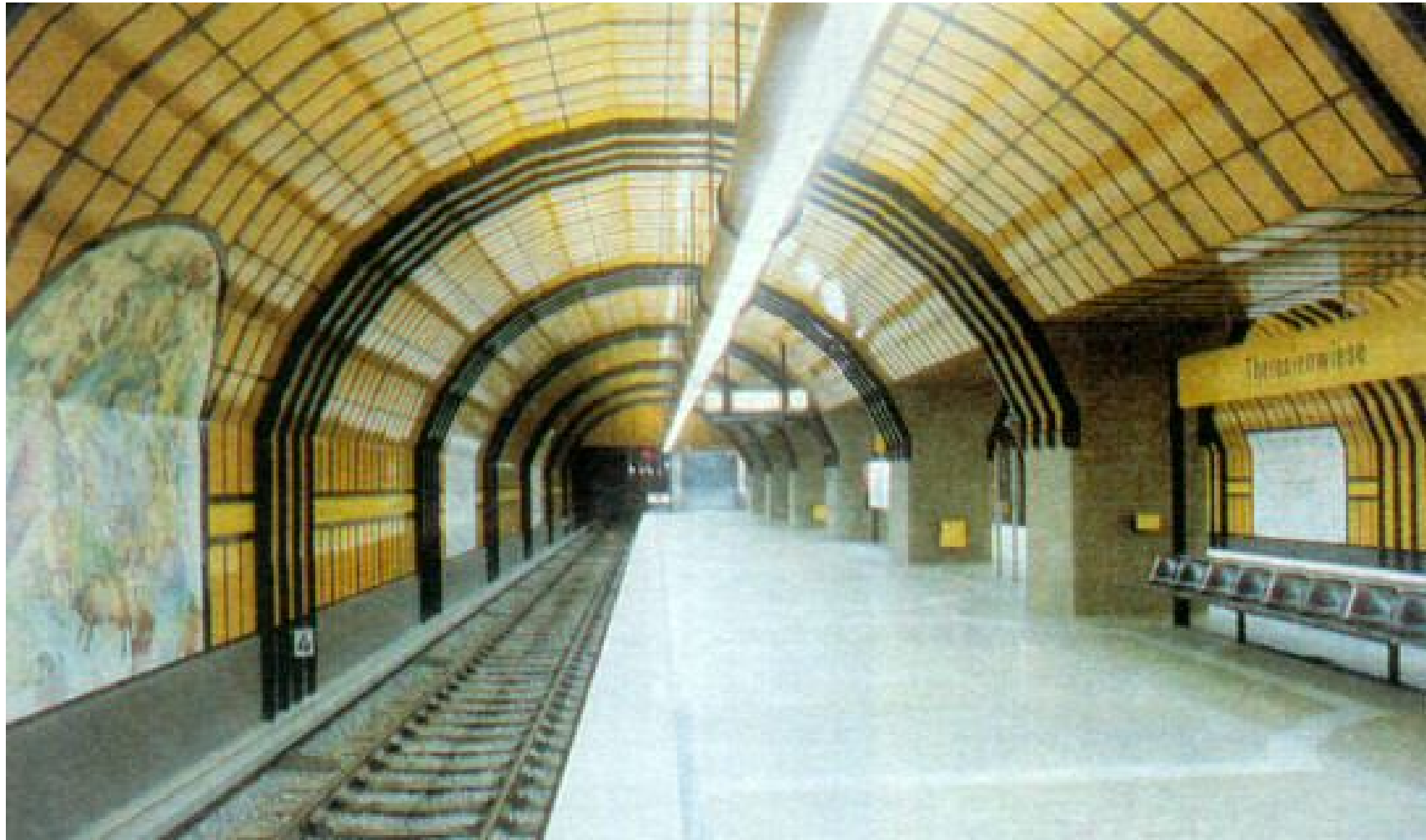
Mined (NATM) Metro Station “Theresienwiese” - Multiple Drift Excavation
