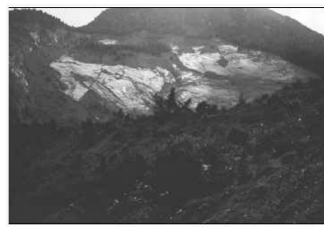
Figure VI-2. View of left reservoir bank following failure
