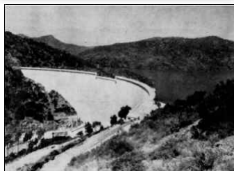
Figure MF-3. Malpasset Dam before failure (after Belier, 1967)
