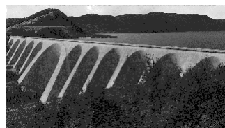
The Daniel-Johnson Dam
