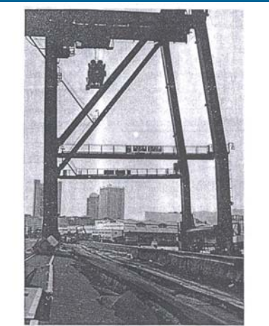
Photo Failure of the Container Berths in Rokko Island
